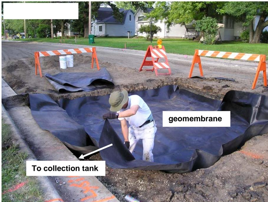
Fig. B1. Installing geomembrane for lysimeter.
