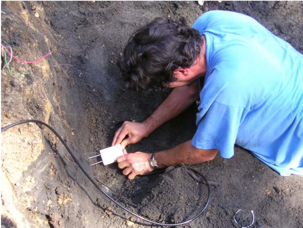
Fig. B3. Installing water content reflectometer in subgrade.
