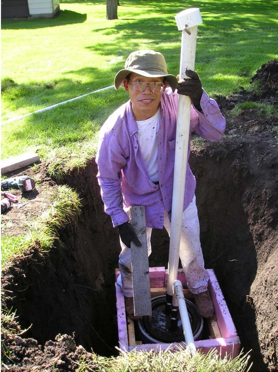
Fig. B2. Installing collection tank for lysimeter.
