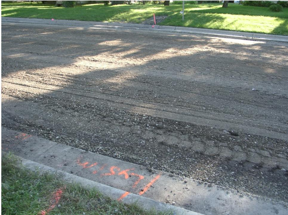
Fig. A1. RPM before placement of fly ash.
